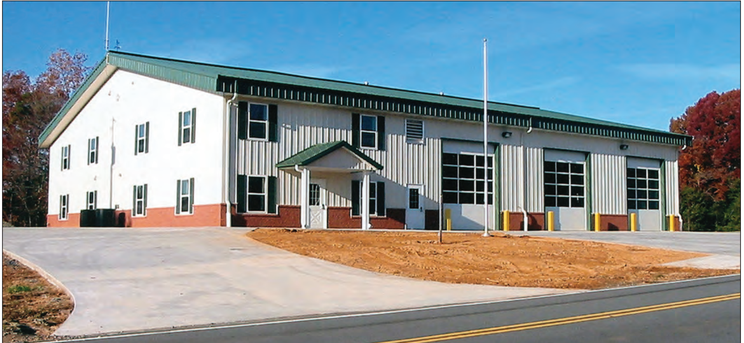
Figure 23. Post-frame allows high sidewalls and wide clear spans for mixed uses.
