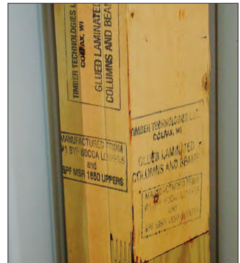
Figure 12. Finger-jointed glue-laminated columns provide one of several good post options. Note treated wood spliced to the bottom end.
