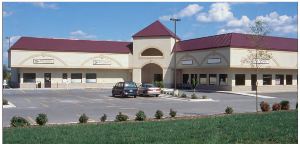
Figure 22. Post-frame is an excellent choice for strip malls and other retail buildings.
