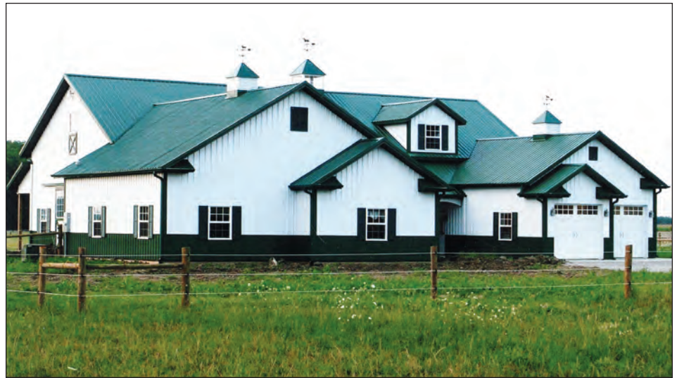
Figure 24. Although any exterior finish may be used, steel siding and roofing are popular due to economy and maintenance-free durability.
