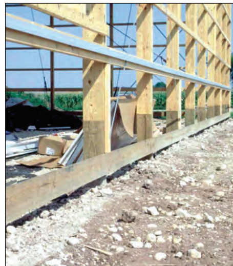
Figure 11. Laminated columns often splice treated wood on the bottom end to untreated wood above grade.
