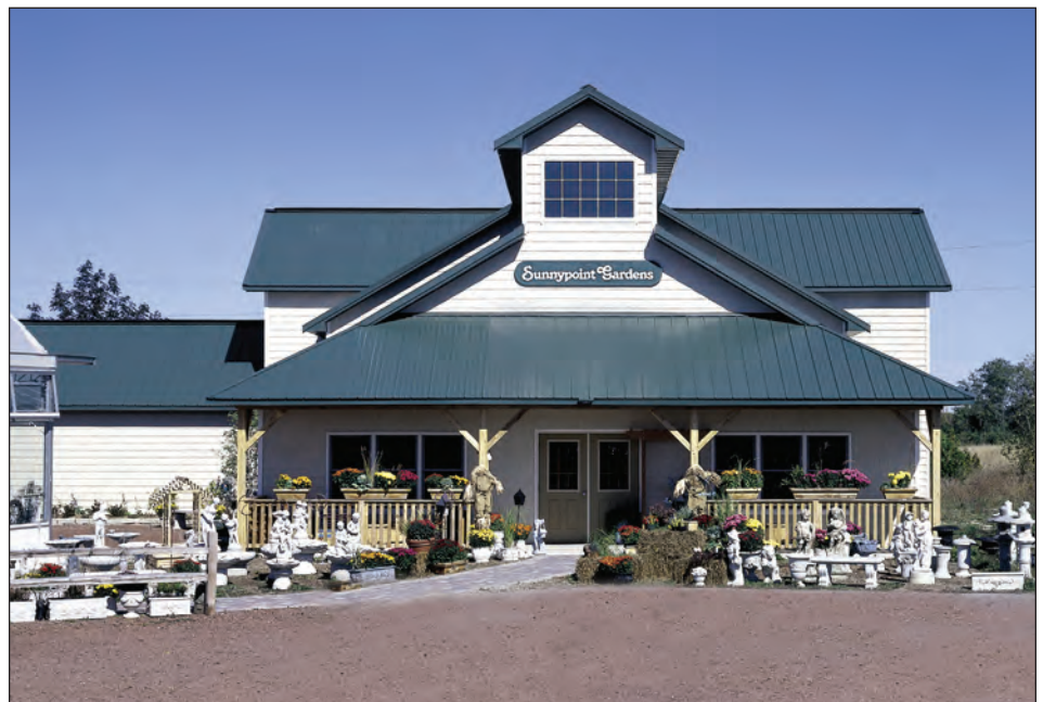
Figure 30. Post-frame garden center featuring retail areas, offices and work areas.
