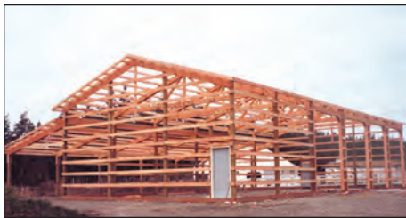
Figure 10. A typical post-frame building frame.
