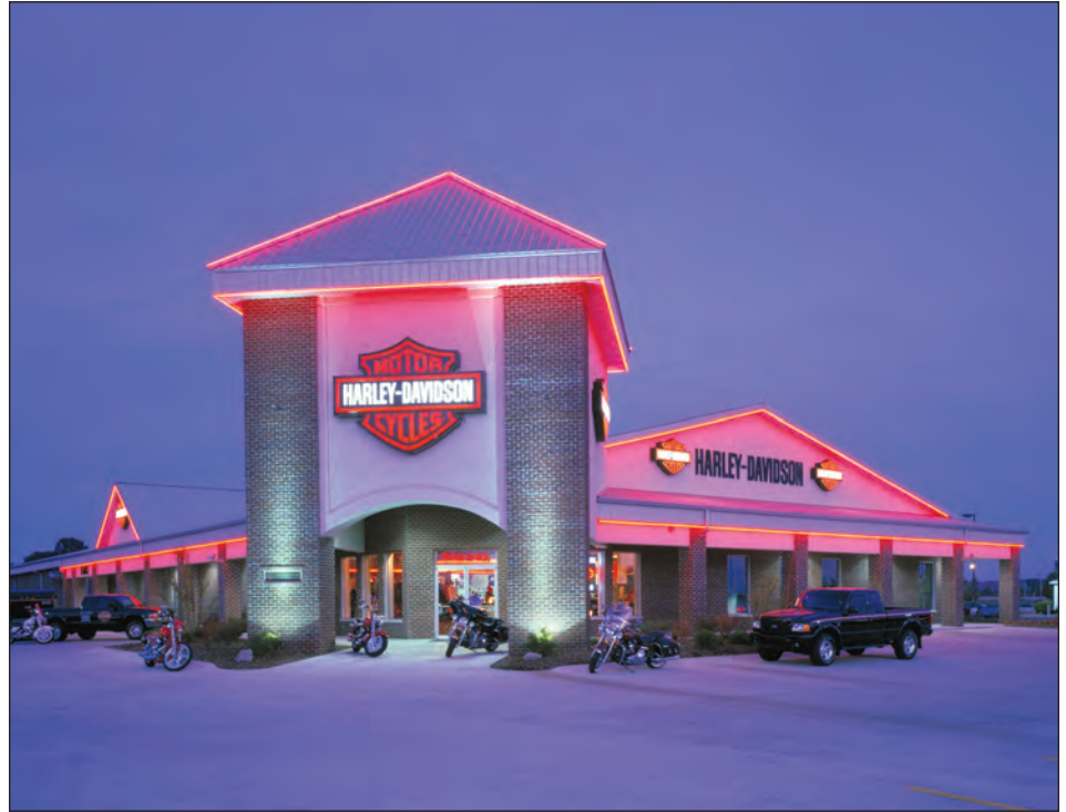
Figure 29. Post-frame retail facility with large interior clear-spans and ample room for show rooms and mechanic's shop.
