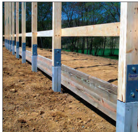
Figure 16. Pre-cast concrete piers provide one of several foundation options unique to post-frame.
